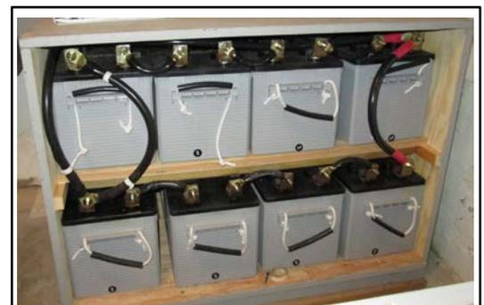
Figure 11. 48-volt battery configuration in a residential application
