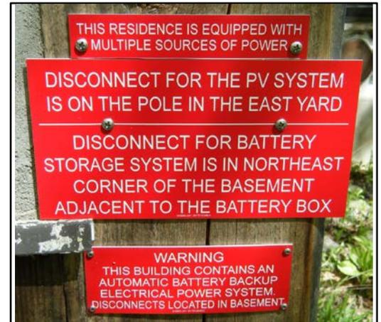
Figure 9. Permanent plaque indicating all power sources on or in the premises
