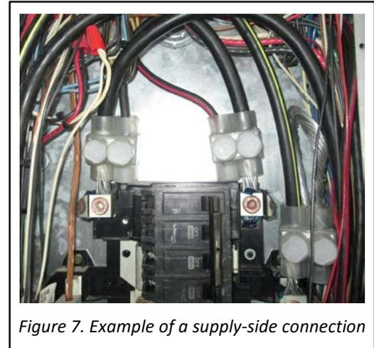
*Figure 7. Example of a supply-side connection*
