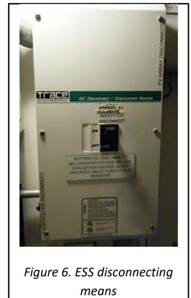
Figure 6. ESS disconnecting means
