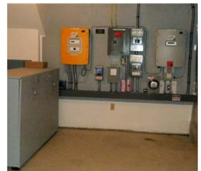
Figure 3. Other energy storage system of individual components
