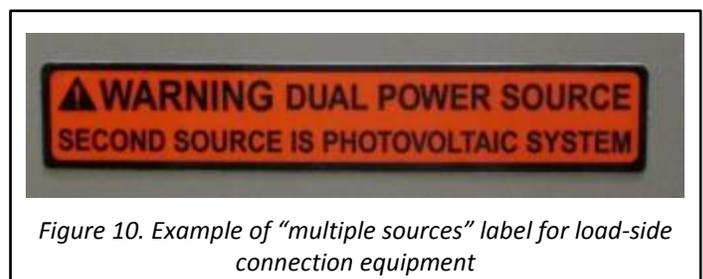
Figure 10. Example of "multiple sources" label for load-side connection equipment
