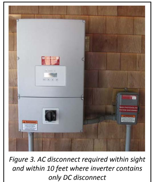
*Figure 3. AC disconnect required within sight and within 10 feet where inverter contains only DC disconnect*
