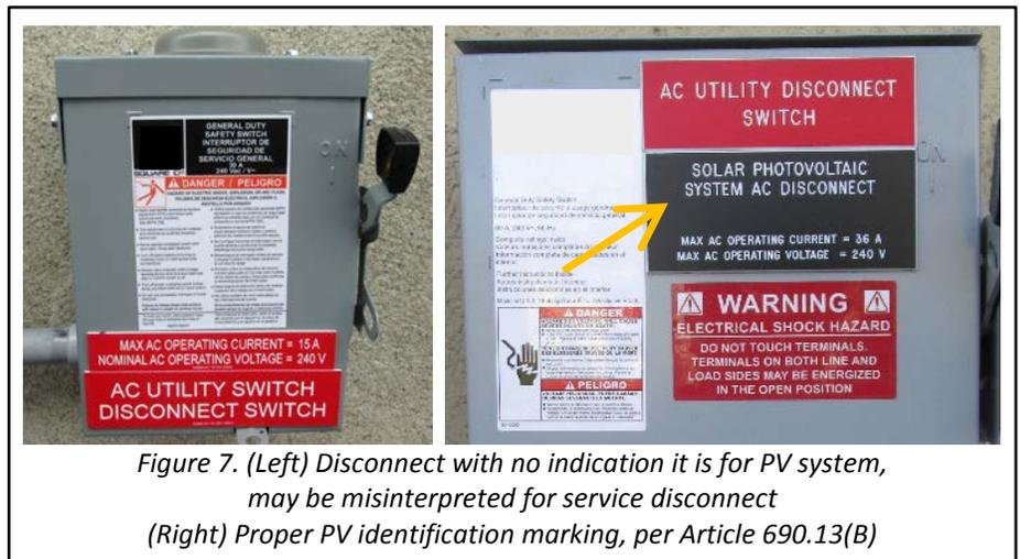
Figure 7. (Left) Disconnect with no indication it is for PV system, may be misinterpreted for service disconnect
