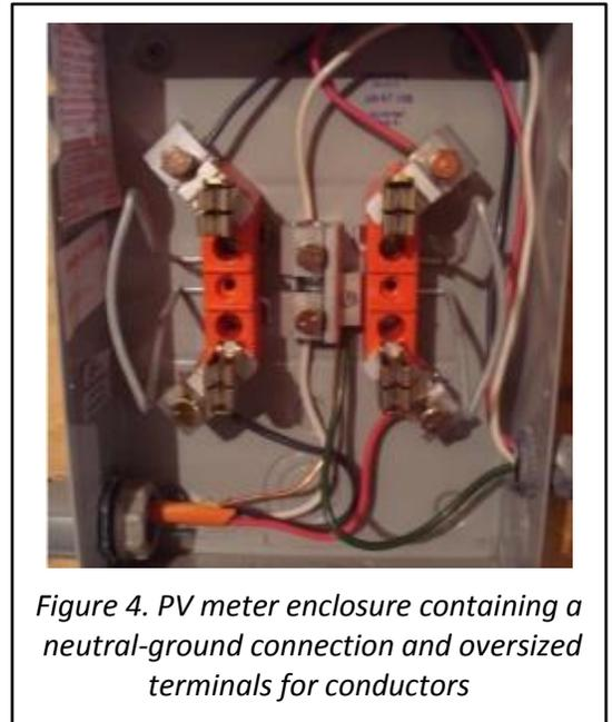
Figure 4. PV meter enclosure containing a neutral-ground connection and oversized terminals for conductors
