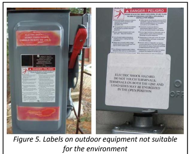
Figure 5. Labels on outdoor equipment not suitable for the environment
