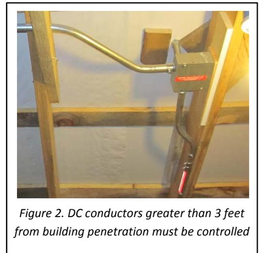
*Figure 2. DC conductors greater than 3 feet from building penetration must be controlled*
