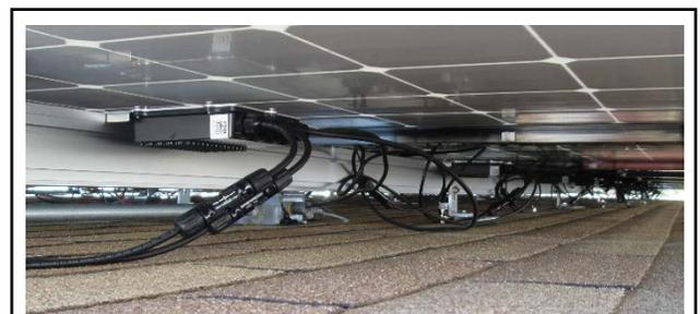
*Figure 1. Conductors below array not properly supported and exposed to physical damage*
